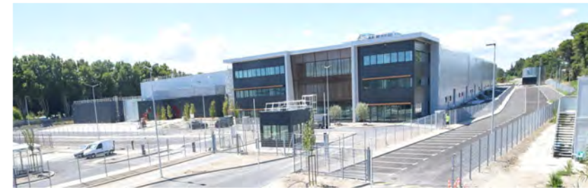
South-East project in Noves
